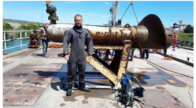
Tempering Water Pump removal
