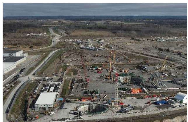
Progress underway for the Darlington New Nuclear Project.
